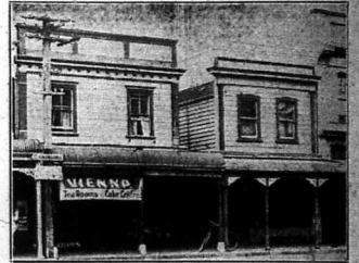
Old Buildings, which were demolished to make way for our New Premises.
