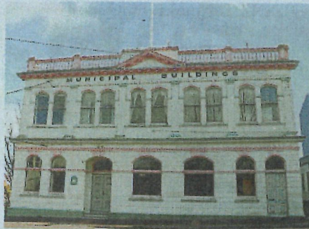
The 1911 Eltham Municipal Building has been closed since 2018.
