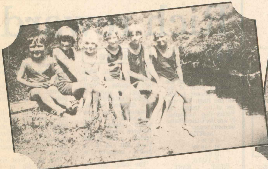
Before the pool work started, it was just a swimming hole . . . (left) Ray Sheppard, Alison Evans, Joyce Sheppard, Nancy Evans, Jean Tippens and Nina Tippens, about 1926. CENTRE: A camping ground was among later developments. RIGHT: The concrete weir outlet for the Huatoki Stream to flow on to the city.
