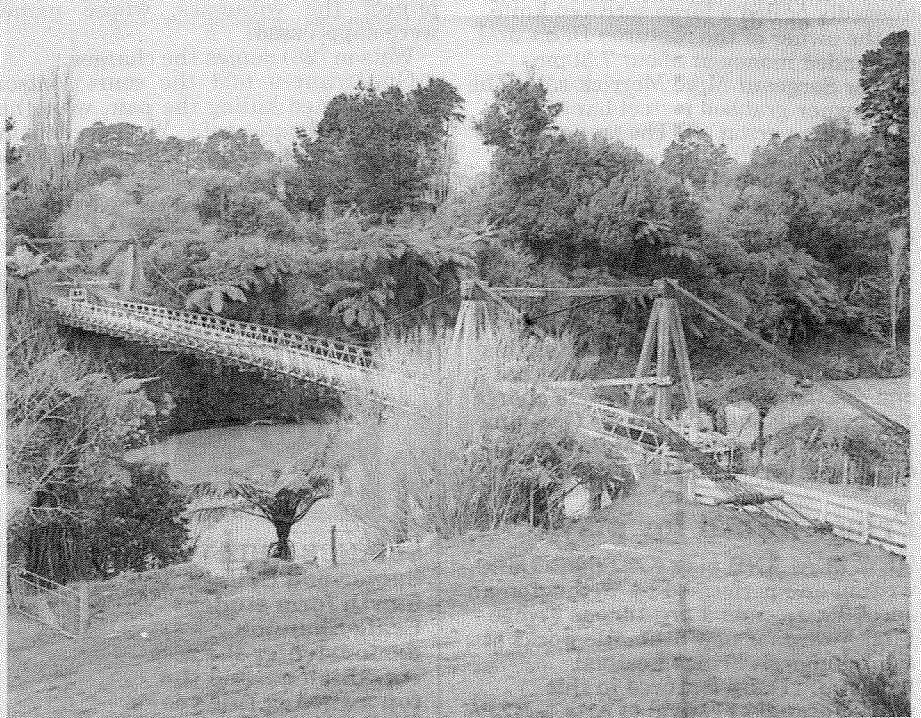
COUNCIL CASH: The historic Bertram Rd suspension bridge was built in 1927, but is now closed to motorised traffic.
