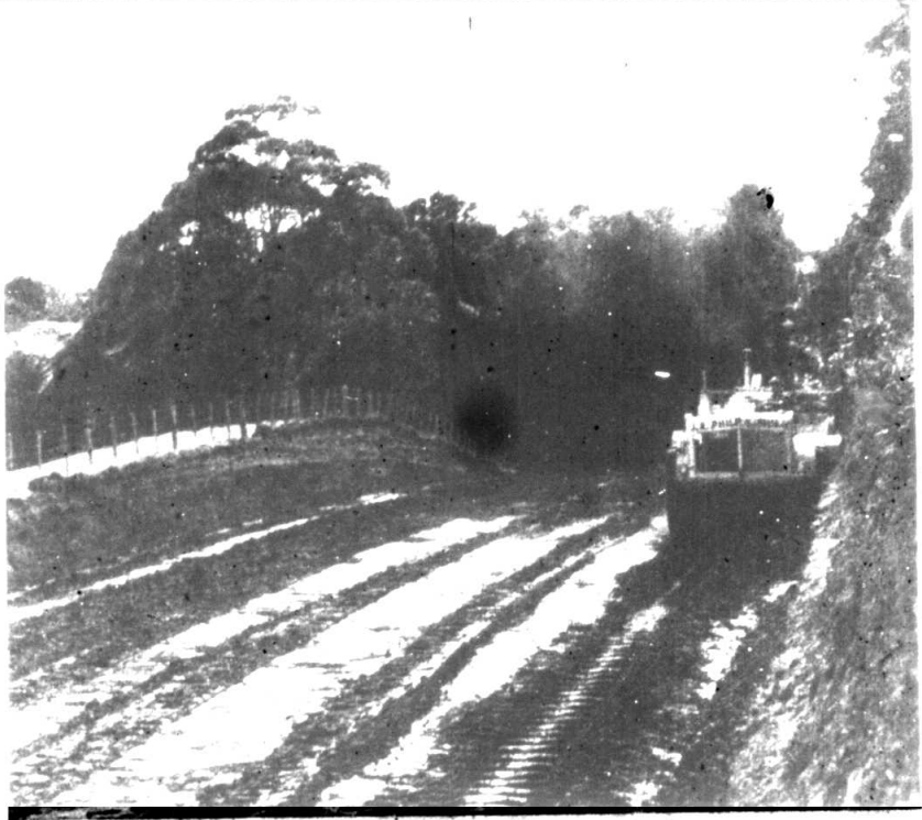
THE FIRST ROADWAY into the Barrett Domain, New Plymouth, takes shape as a huge earthmoving machine scrapes tons of soil off the top of a hill for filling over a culvert in the Mangaotuku Stream. The earthworks for a quarter-mile of road at the Roto St entrance were expected to be completed today.
