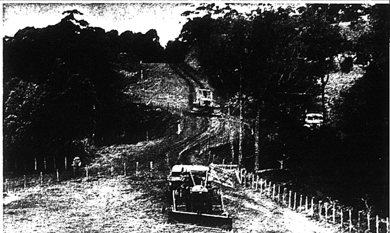
BULLDOZERS move in to start work on completing the road access to New Plymouth's Barrett Domain. The new work will start at the culvert (centre) over the Mangaotuku Stream and continue to the Barrett Lagoon.
