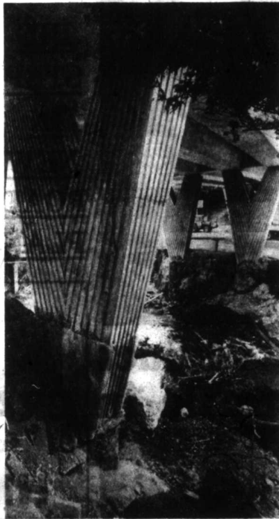
Massive reinforced concrete piers, part of the support structure
