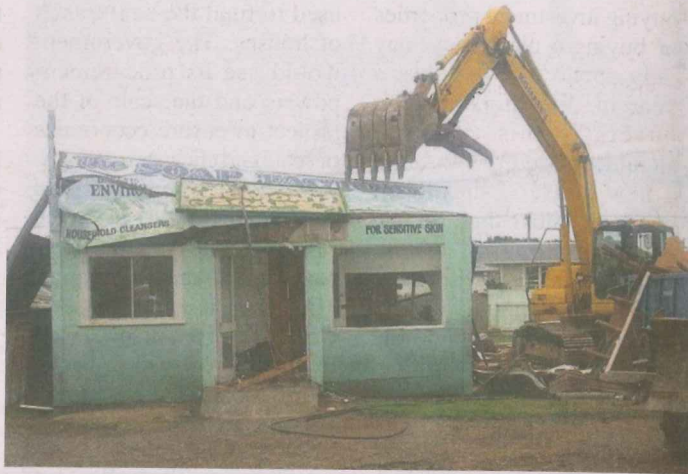
Egmont Soaps factory being pulled down recently.
