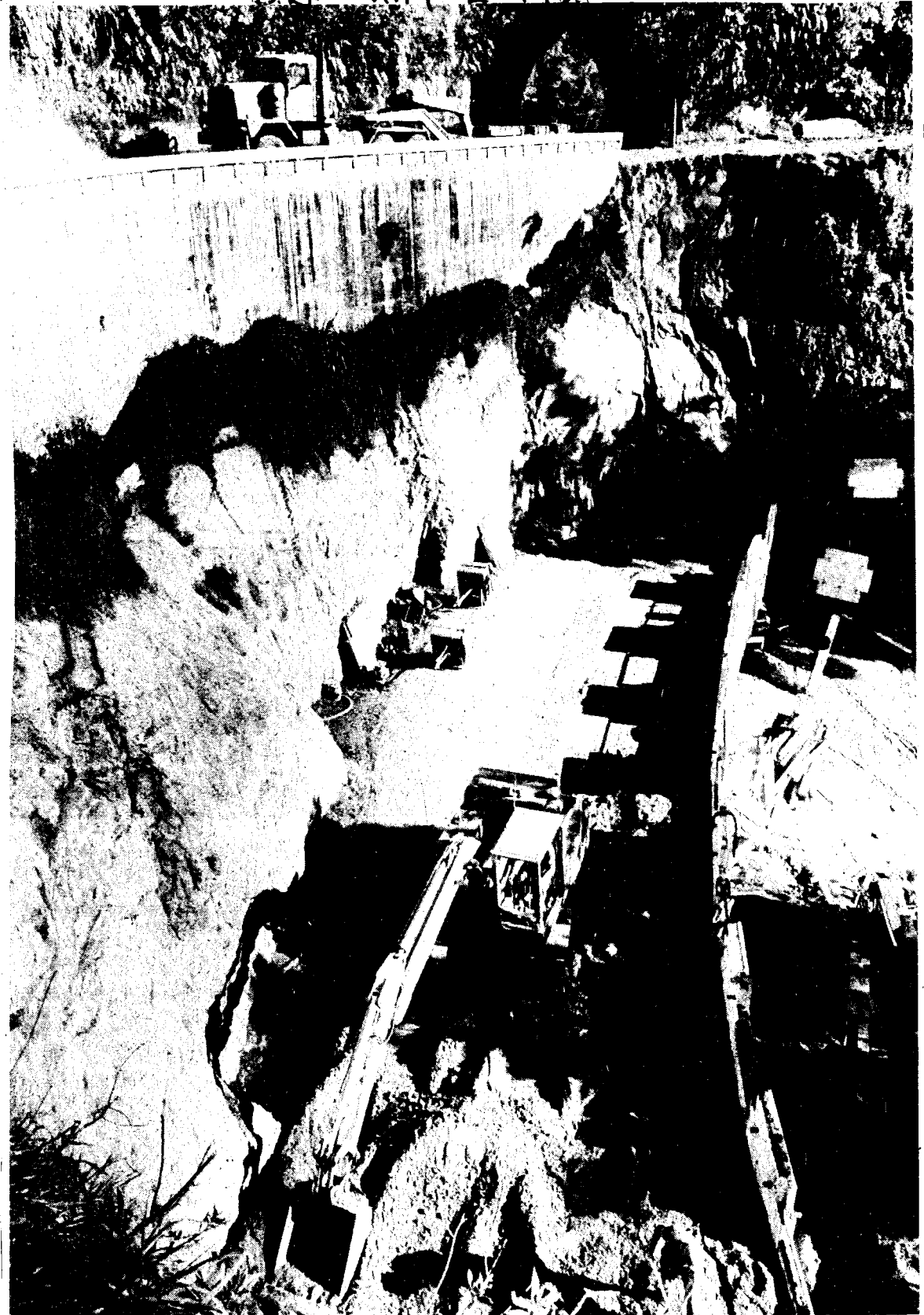
Road and tunnel widening at this point (above) on Mt Messenger is running two to three weeks behind schedule — and motorists may be delayed between 8am and 5pm daily — because of unusually hard earth which needs to be removed in the area. A retaining wall has had to be built after massive excavations. The existing road will be dropped about 2.5 metres to create a new road, including that now being filled. The tunnel is also to be widened.
