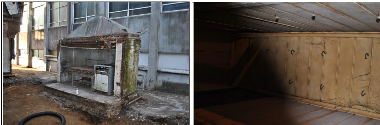
Plate 10: (Left) Kitchen Fireplace following the removal of the kitchen addition - dating to the 1887 rebuild. Plate 11: (Right) Ceiling hooks and a match lined ceiling, noted in the passage to the kitchen in the 1901 Messenger plans.
