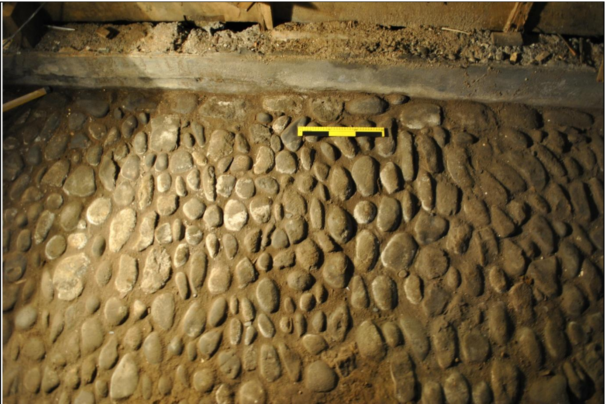
Plate 22: Detail of cobbled floor, concrete foundation at top of shot is the northern wall of the 1887 building
