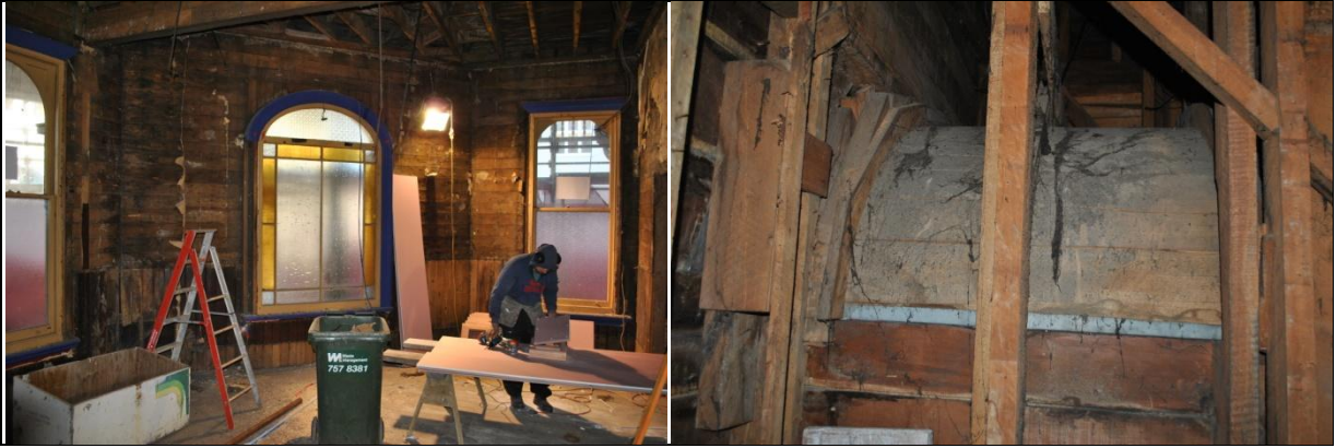
Plate 12: (Left) Ground Floor corner window, installed in place of the corner entrance to allow for the ground floor sitting room in the 1901 Messenger extension. Plate13: (Right) Interior of the vaulted ceiling of the Devon St entrance, exposed during interior re-cladding.
