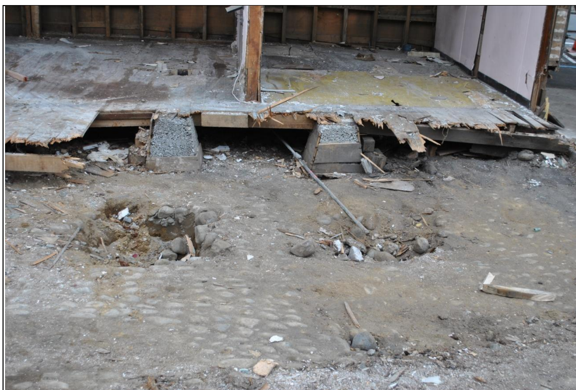
Plate 25: Beach shingle concrete piles, two standing, two removed, boxing still attached
