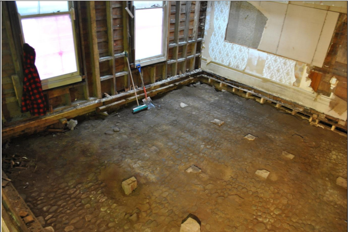
Plate 18 Cobbled floor and protruding piles, photographed in dining room following the removal of floorboards
