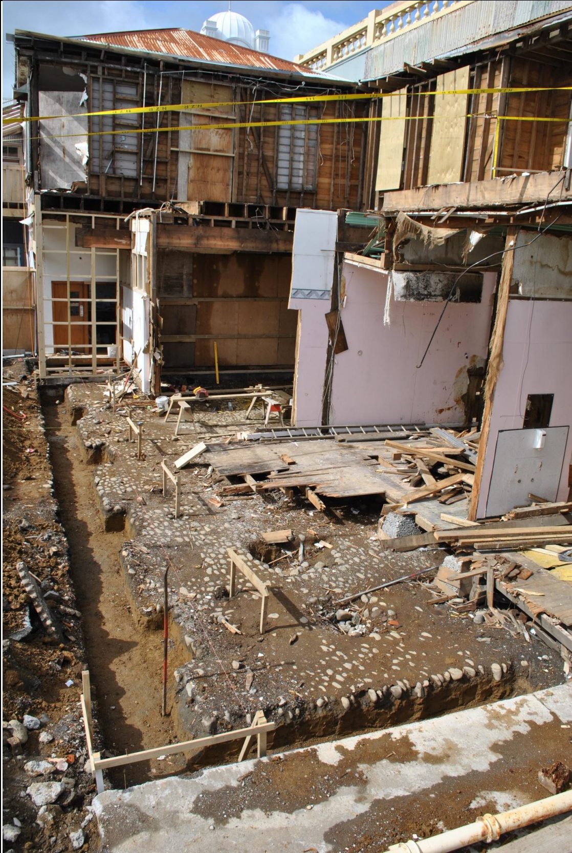
Plate 20: Ring foundation cut through the cobbled courtyard, which remains otherwise intact
