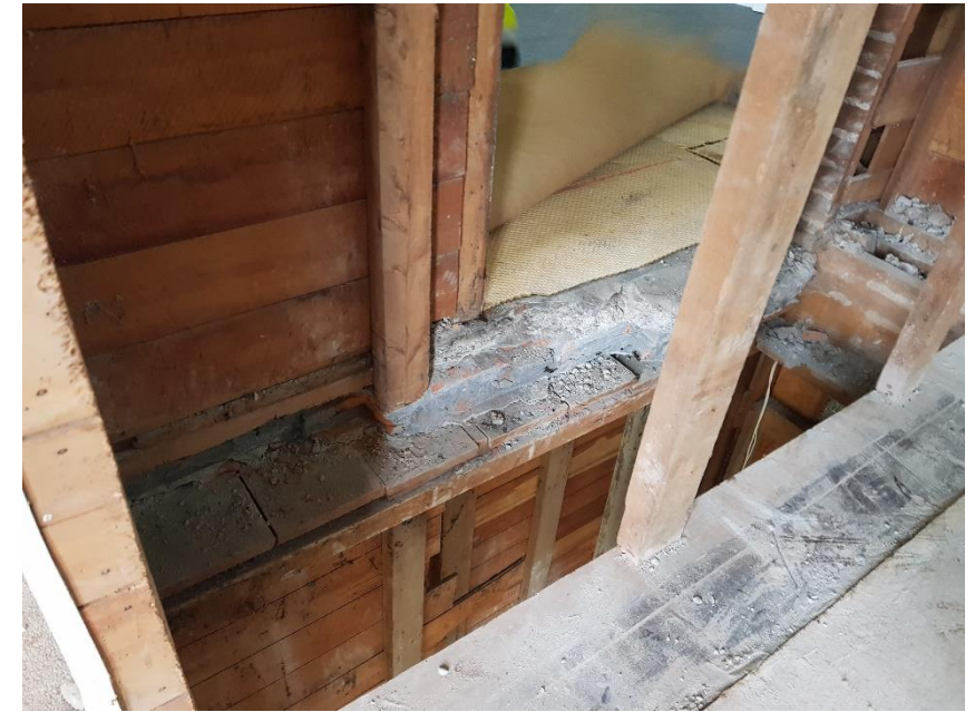
Upstairs Bedroom 4 fireplace (after removal)
