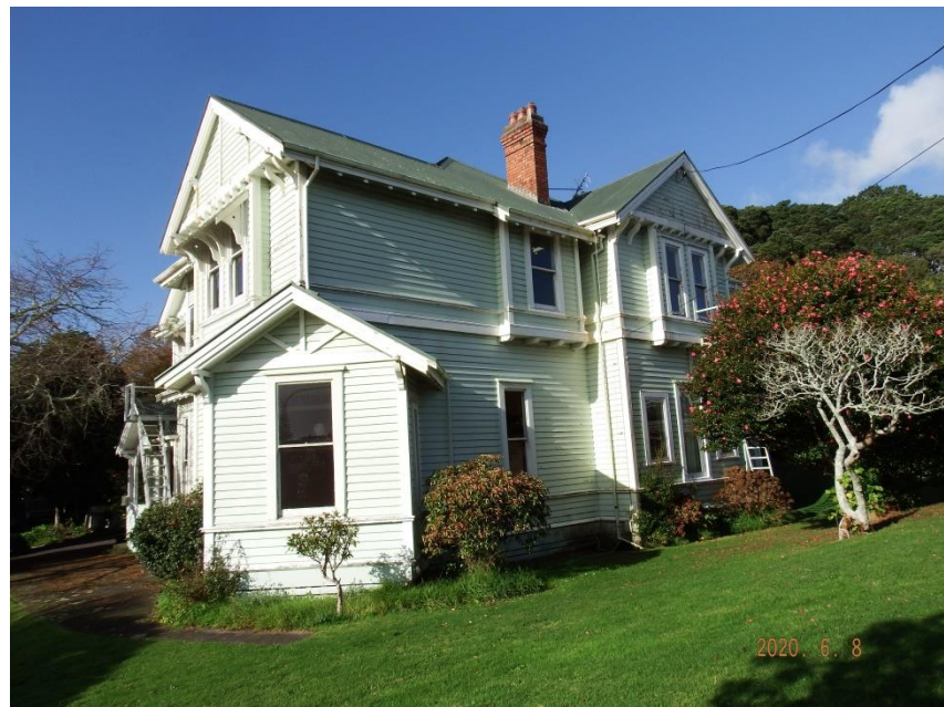
North West view
