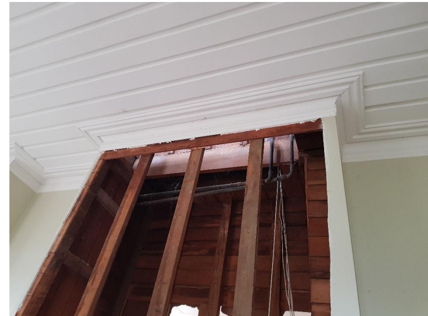
Fireplace (after removal)
