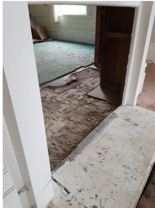
Lounge fireplace (after removal)
