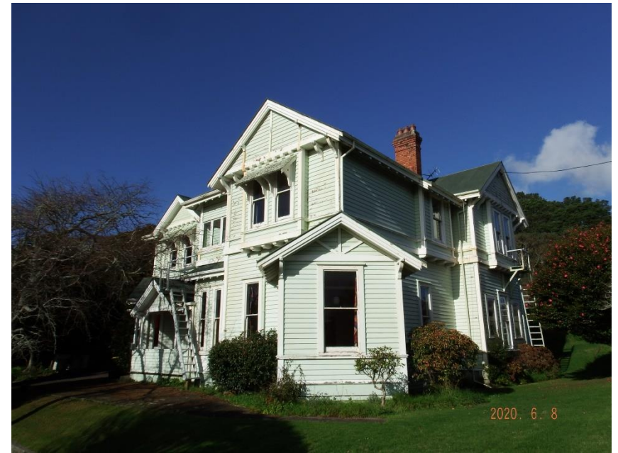
North West view
