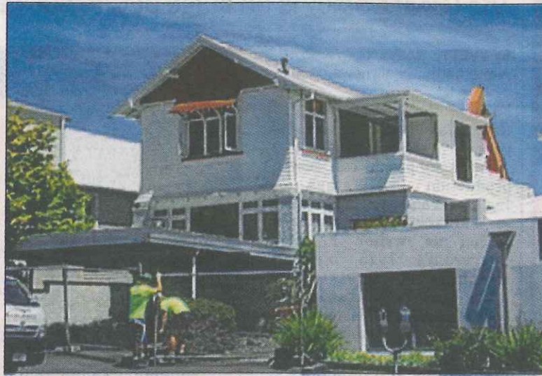
Demolished: This two-storey timber and roughcast building on Robe St was pulled down on February 9 to make way for the new police station. It was built in the 1920s as a private home for the Hooper family and designed by Frank Messenger, who played a part in alterations to the White Hart hotel.
