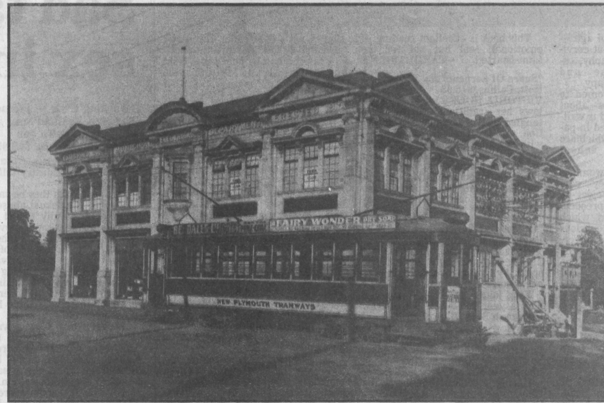
The original New Plymouth Municipal Electrical Department Building doing the job it was built to do . . . converting power to run trams. This photo pre-dates its extension in 1936.
