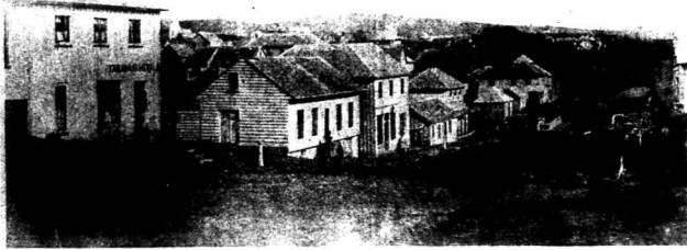
Above, the Herald's first home in 1852 on Devon Street. Below, larger premises in Devon Street until 1900.
