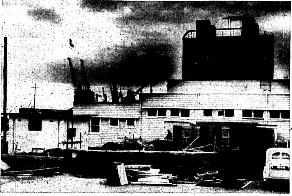
WORK has started on the new Taranaki Harbour Board office at the New Plymouth Port. This photograph, taken from near the port weighbridge, shows preparations being made for the laying of foundations. The site is dwarfed by the waterfront Industry Commission building and the cement silos in the background. The Newton King Wharf cranes are shown in the left background.
