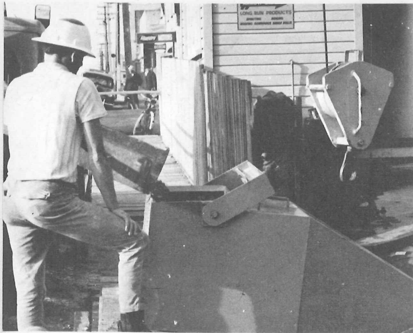
Above : Cement hoppers with ready-mixed cement pull up on the side of the site, where it is transferred into the hopper of the crane and transferred to the part of the job where required, by right, the operator who walks around with his small control box to any part of the building site. Below, left : This is how the new crane looks from below. Below, right : Very little space is required for the base of the crane in the basement of the building.
