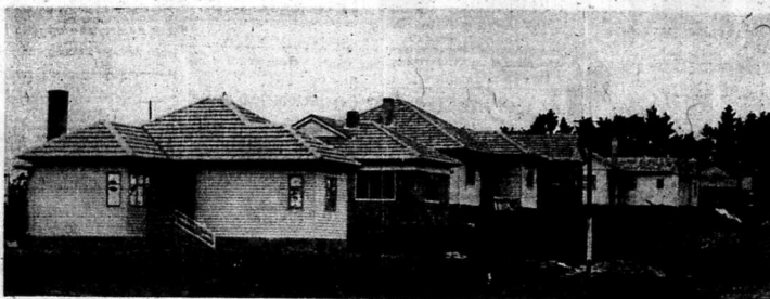
A general view of the first group of State houses at New Plymouth, many of which are now ready for occupation.
