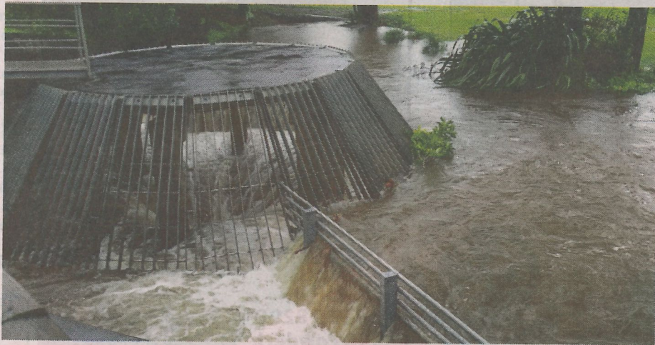
The "roaring" water at the Bonithon Avenue diversion tunnel during the storm.
