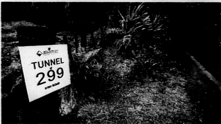
The condition of the road deteriorates after the tunnel. The council has an option to eventually close the rest of the road.
