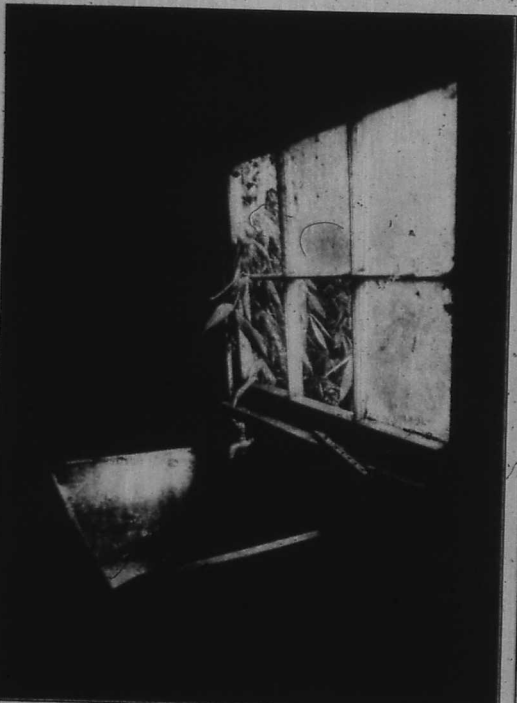
WASHED OUT: The original kauri tubs in the washhouse, at the back of the house, have seen better days.
