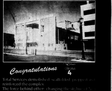
Congratulations Total Services demolished, scaffolded, prepared and reinforced the complex. The force behind other changing the skyline of New Plymouth — GOOD ONE MARTY! Thanks ... Graham Harris Ltd for concrete breaking and the removal of spoils.
