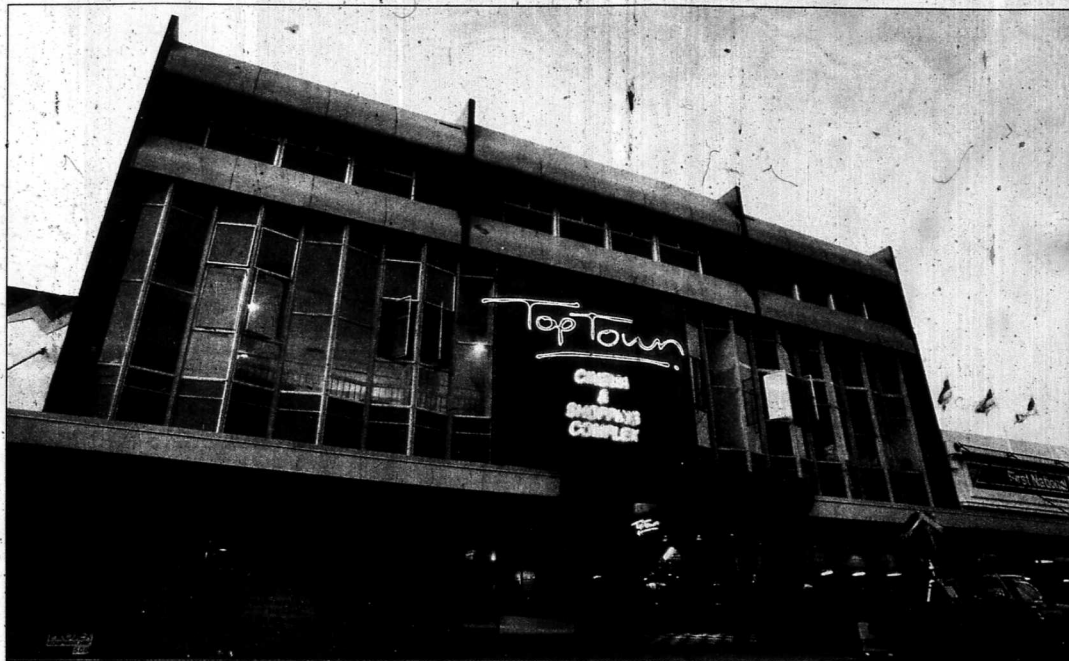
TOP TRANSFORMATION: The colourful, brightly-lit exterior of the new TopTown Cinema 4 complex in New Plymouth is light-years away from its former appearance as the city's Farmers' Co-op department store. Photo: DWAYNE SENIOR
