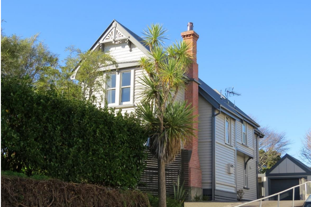
Front gable and south-western side elevation
