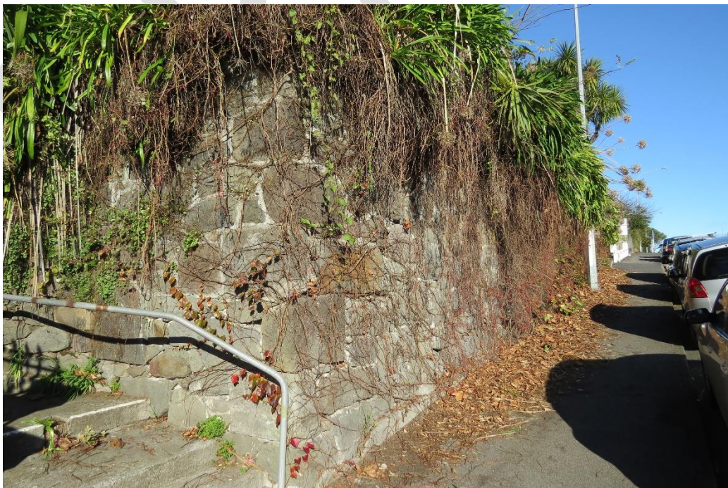
Looking west along andesite retaining wall
