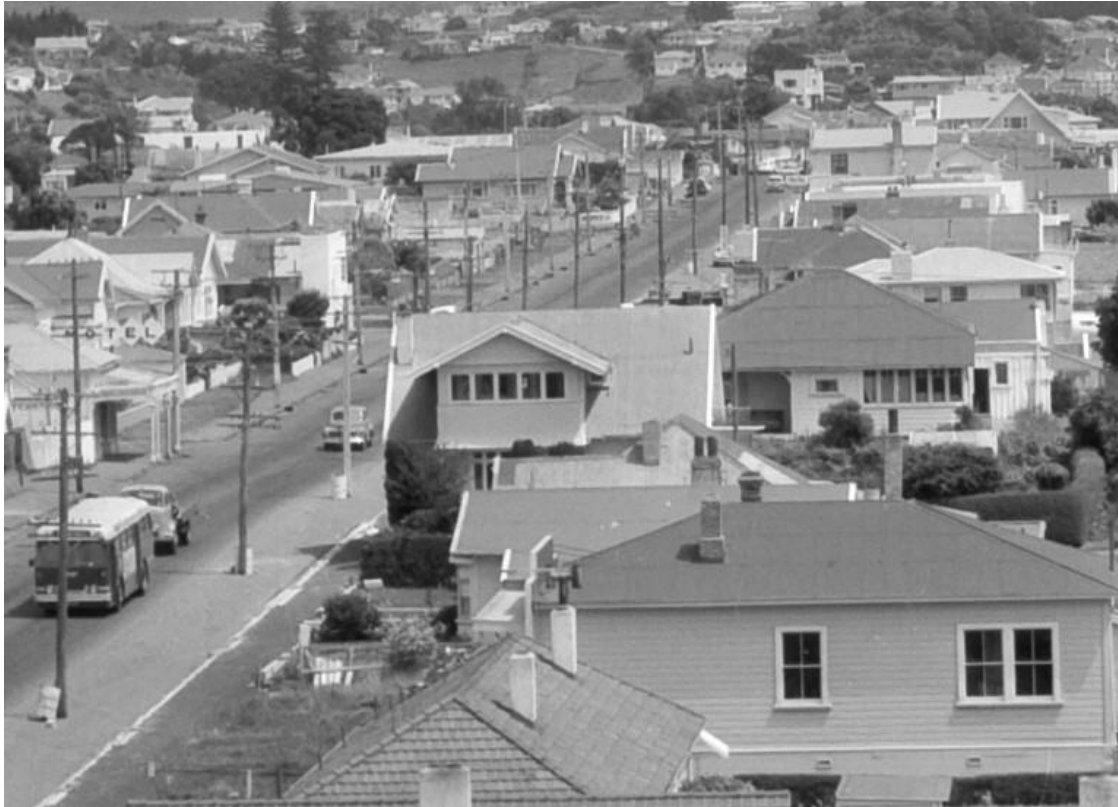
Detail showing 162 St Aubyn Street from photo of New Plymouth looking west from Tasman Hotel/Richmond Estate – note the recent street widening with power poles yet to be shifted to their new positions, 16 th February 1965, Whites Aviation, Alexander Turnbull Library, WA-63531-F
