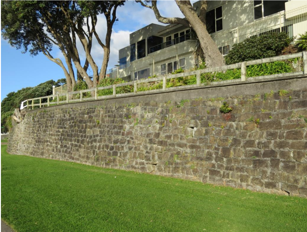
Retaining wall looking east towards playground area
