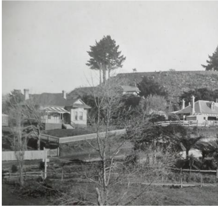
Detail from circa early-1898 view of Vivian Street looking south-east towards Marsland Hill, by George Herbert White. House still in single storey form and stone retaining wall yet to be constructed. Puke Ariki Collection, A.3.24
