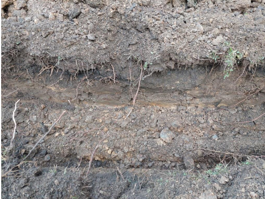
Figure 13: Crushed rock and clay material uncovered during excavations for the stormwater pipe trench in the vicinity of the NPDC sewer line installed circa 1979 (Hamish Crimp, 16 May 2022).
