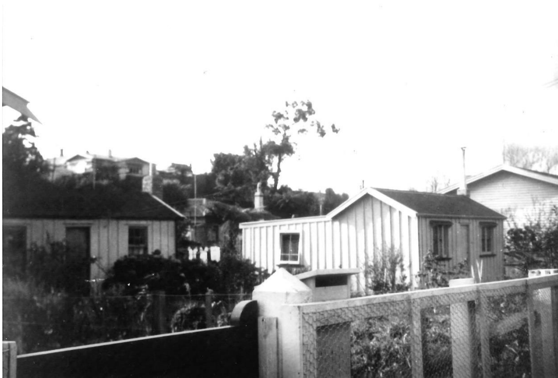
Figure 6: Photograph taken some time between 1933 and 1966 showing 4 (at right) and 6 (at left) Aubrey Street close to their original form. 6 Aubrey Street has been shifted back on the section, but still retains its original board and batten cladding and twelve-light sash windows. The Puke Ariki record notes these as being the 65 th Regiment Quarters. (65 th Regiment Quarters, Aubrey Street, Puke Ariki, PHO2006-333).
